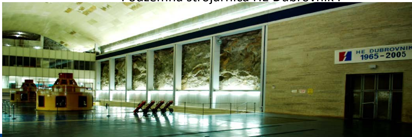
Podzemna strojarnica HE Dubrovnik I
